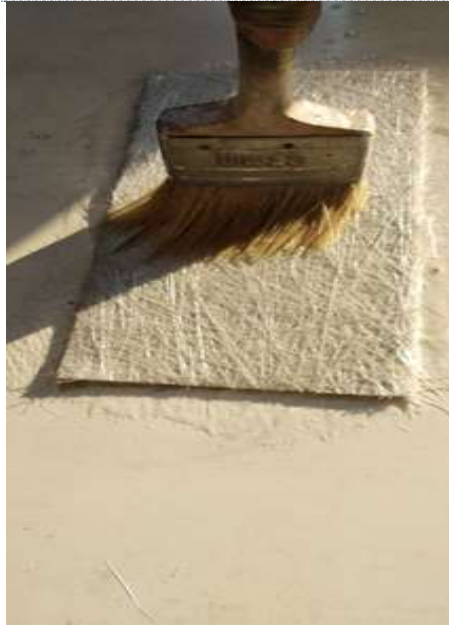
Fig 2. Application of epoxy on chopped Glass fiber sheet
